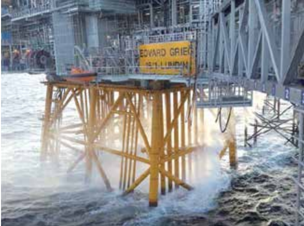
Figure 15. For the Edvard Grieg platform jacket, Dillinger delivered 12,400 tonnes of thermomechanically rolled steel of the grades S355G10+N/+M, S420G2+M and S500G2+M.
