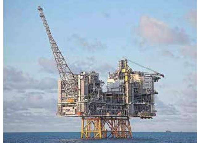
Figure 16. The 22,500 ton topside module of the Edvard Grieg platform, which is equipped with highly complex technology, 100-person living quarters and a helicopter deck, is built on a foundation structure made of Dillinger steel.
