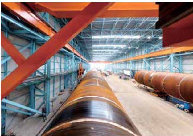
Figure 9-10. At the Roermond site, the large shell sections are assembled into XL monopiles.
