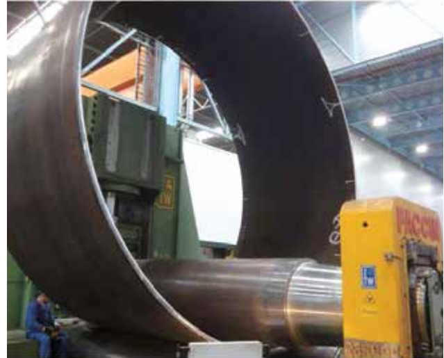
Figure 5. After each welding process, the shell sections, which are up to 11 meters in diameter, are calibrated in a ring roller.
