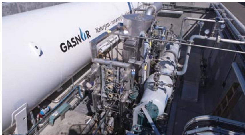
FGSS developed independently by DSME
