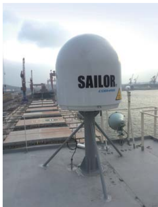
Installation of SAILOR 900 VSAT antenna on deck
