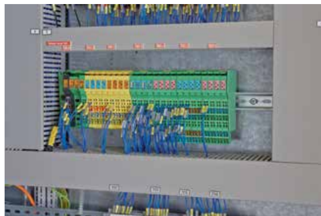
Figure 5. As part of the Inline station, the safety-oriented modules are used to control and monitor the four lift bridges and the corresponding gate systems.
