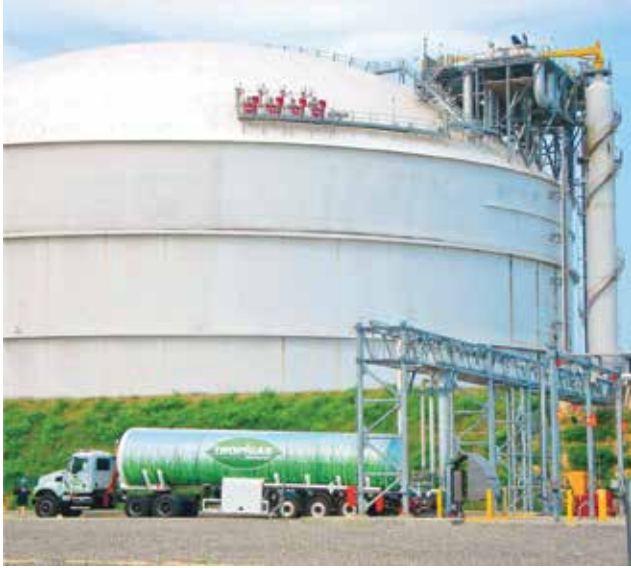
Figure 6. LNG is loaded into distribution trucks at the AES LNG import terminal in the Dominican Republic. The large 160,000 m 3 LNG tank in the background is an atmospheric pressure tank with a reliquefaction system.
