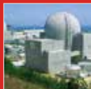
Nuclear Power Plant Cable
