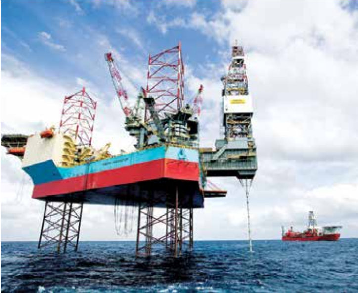
Bird's eye view of the large jack-up rig ordered to DSME
