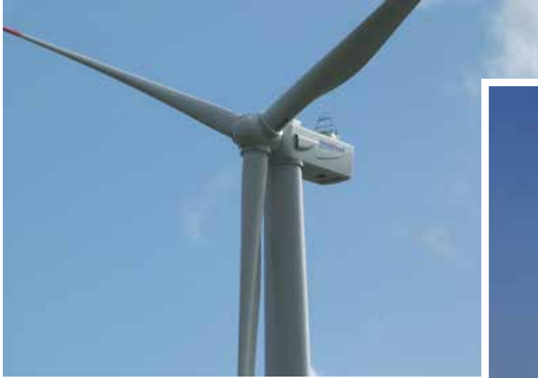
Figure 6. 'D 9.1', the 2MW wind turbines which DSME will supply to the wind farm in Hasa-ri
