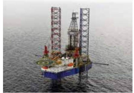
(Source: Vantage Drilling)
