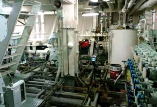
Scanning the Engine Room onboard a ship with the Focus 3D
