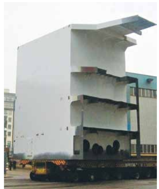
Figure 3. The new funnel casing structure ready to be lifted on board.
