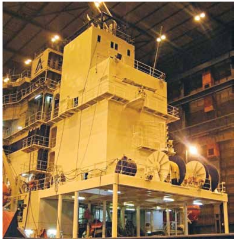
Figure 5. The new funnel casing installed on the deck extension.
