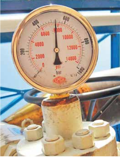
Figure 9. Pressure testing of the gas pipeline.
