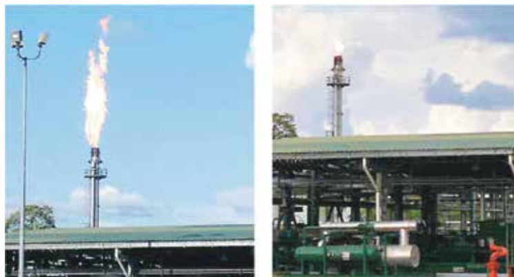
Figure 5~6. Gas Flaring at Eden Yuturi before and after the GD conversion.
