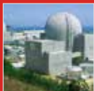
Nuclear Power Plant Cable
