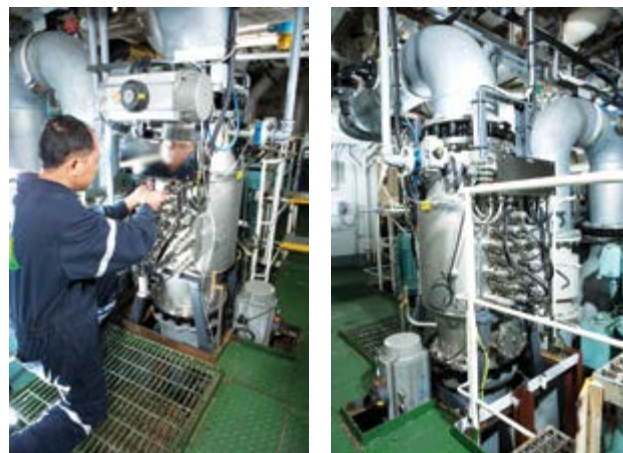
Figure 4. PureBallast 3.0 system onboard: The smaller number of units in most configurations of PureBallast 3.0 means that considerably less pipework is required.
