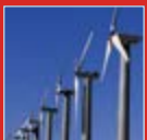
Wind Turbines Cable
