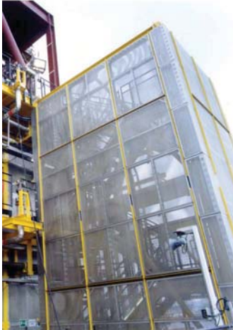
Figure 4. Darscreen wind shield for offshore platform stairway
