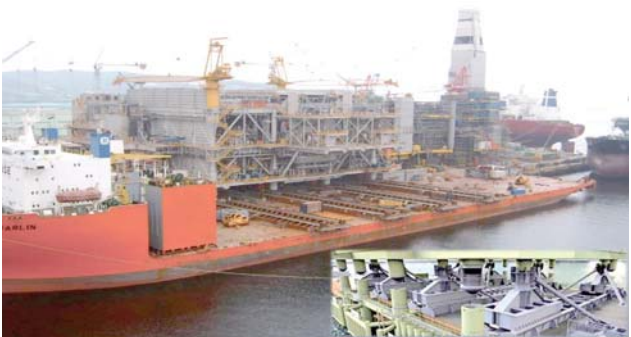
Project Name: OFON 2 T&I Client: Technip Project Description: Substructure & Grillage for Load out of OFON 2 Topside Construction Scope: Sub-structure & Grillage Modification, Refurbishment
