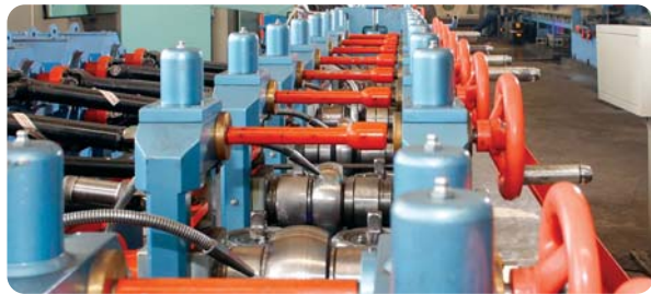
Deploy advanced controllers to optimize existing equipment
