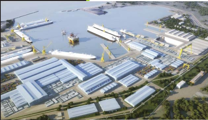
Zvezda-DSME shipyard is the joint venture formed between USC (United Shipbuilding Corp.) and DSME, located in Vladivostok, Russia.
