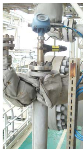
Emerson's Rosemount Guided Wave Radar enables accurate and reliable level measurements in challenging process conditions on the FPSO.
