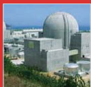
Nuclear Power Plant Cable
