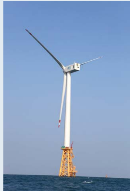
3 MW offshore wind power generation system of Doosan Heavy Industries
