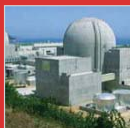
Nuclear Power Plant Cable
