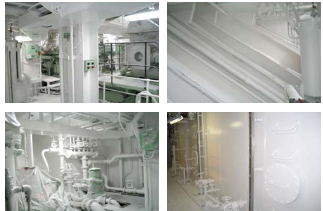
Figure 12. NPMK is the first company that introduced 'Odemarine PF' (Engine Room, Machinery Space), the water-based coating which dramatically reduced VOC emissions, to Korea.
