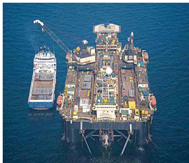
WINGAS relies on RMG by Honeywell for precise metering in the Nord Stream underwater natural pipeline project.
