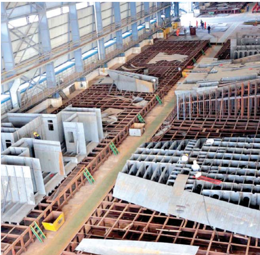
Blocks under construction. Photograph courtesy of PaxOcean Engineering.
