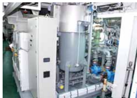
Figure 6. 'HiBallastp', developed independently by HHI last year, filters out various aquatic organisms larger than 50 μm from the seawater inside the ship's ballast tank and sterilizes them through electrolysis.
