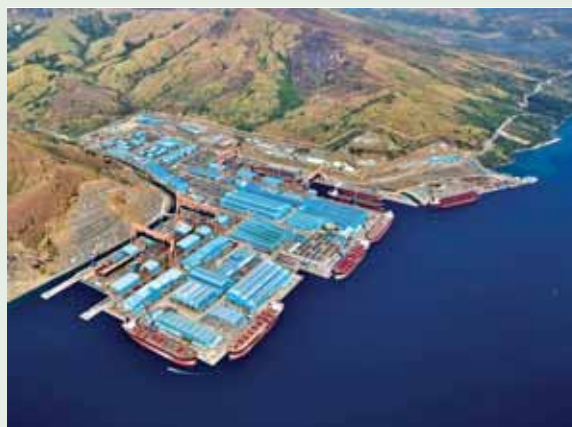
HHIC-Phil's Subic Shipyard, completed in 2009, was built on 800,000 pyong of land in Subic Bay and is equipped with the world's largest dock measuring 550m in length and 135m in width, 4km-long quay wall facilities, 4 goliath cranes and automation equipment.
