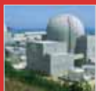
Nuclear Power Plant Cable
