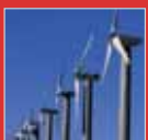
Wind Turbines Cable
