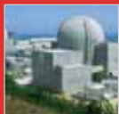
Nuclear Power Plant Cable
