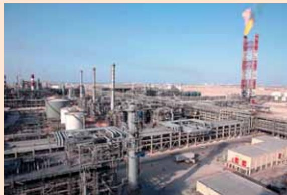
GTL plant in Ras Laffan, Qatar, completed on November 22 by 12 international construction and engineering companies including HHI
