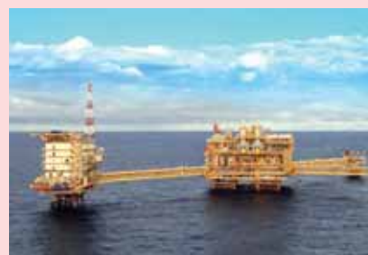
A facility similar to the gas platform awarded to HHI this time, which is the Bongkot gas platform installed by HHI this year in Bongkot oil field in the sea off the southeastern coast of Thailand
