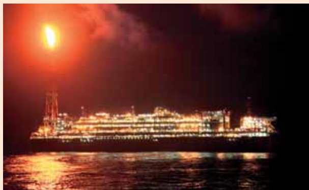
Pazflor FPSO which successfully produced 1st oil in Angola
