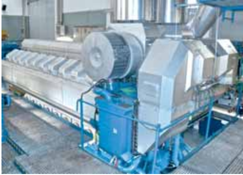
A Wärtsilä 4-stroke diesel engine with two stage turbocharging technology.
