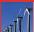
Wind Turbines Cable
