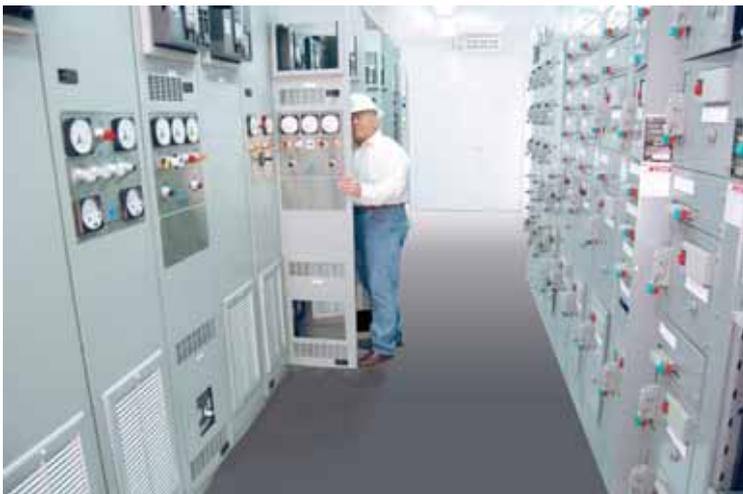
AC drives (VFDs) are now recognized as the preferred method of control for offshore and land rig equipment. AC drives provide many benefits over old technologies including better control, faster block speeds, lower fuel consumption, enhanced drilling and tripping operations, and lower maintenance costs.
