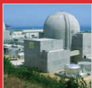
Nuclear Power Plant Cable
