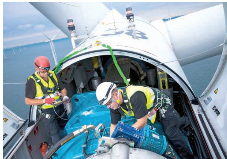
Fig. 2 Installation in the pod of a wind turbine
