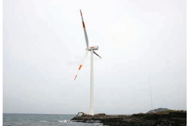
Wind turbine in Wolryeong-ri, Jeju province, which has been in commercial operation by STX Energy since July last year
