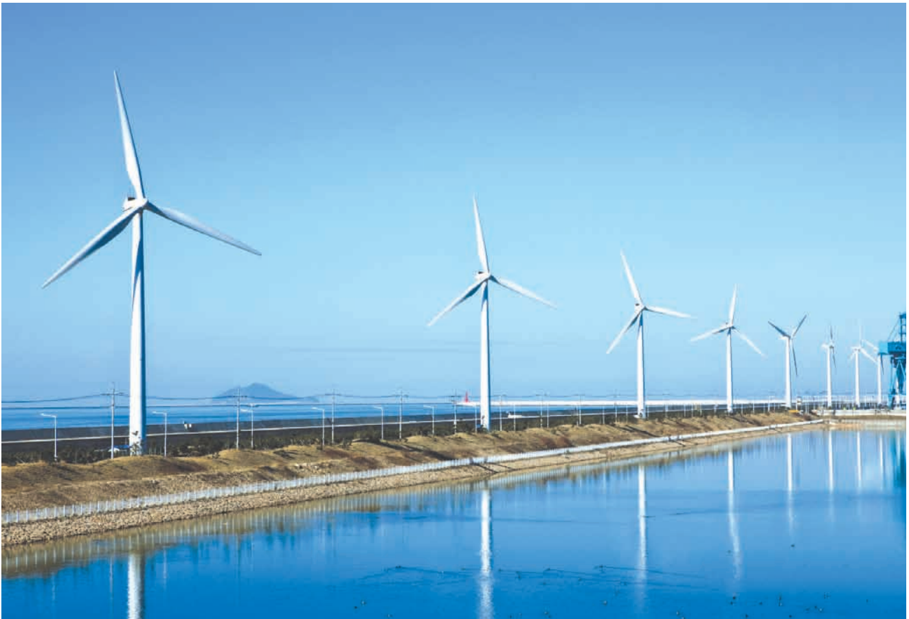
Wind turbines installed by STX Heavy Industries in Saemangeum Industrial Complex
