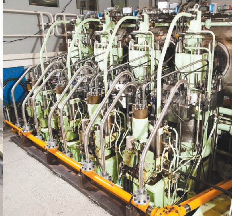
High Pressure Fuel Gas Supply system (left), developed independently by DSME, and MAN Electronic Gas-Injection Engine (right) of MAN Diesel & Turbo
