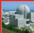
Nuclear Power Plant Cable
