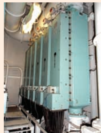
Installation of Electro-Clean System
