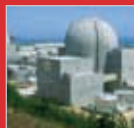
Nuclear Power Plant Cable
