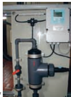
Waterpilot FMX167/ Level measurement in fresh water tank
