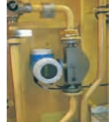
Promass E as oil counter in the supply pipe to the engine
