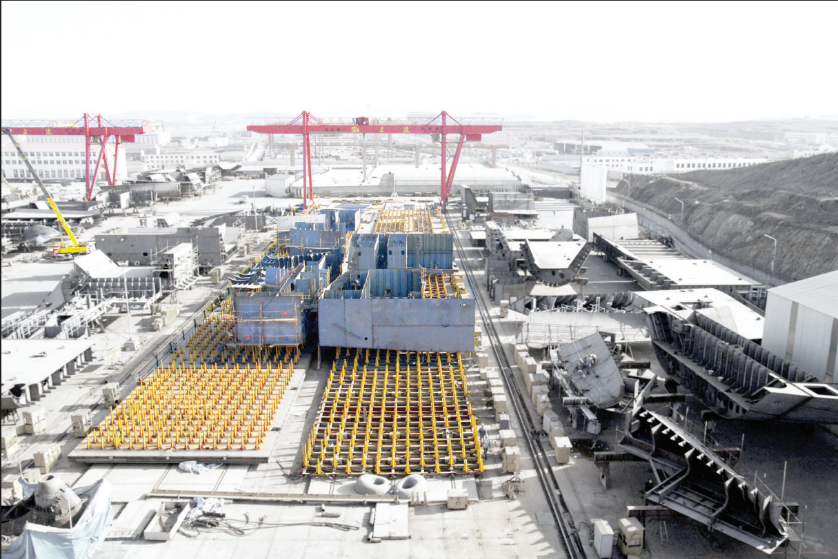
Outside view of the No. 3 factory
