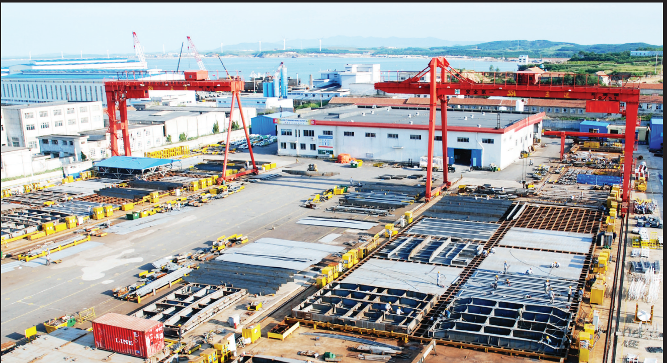
Outside view of the No. 2 factory
