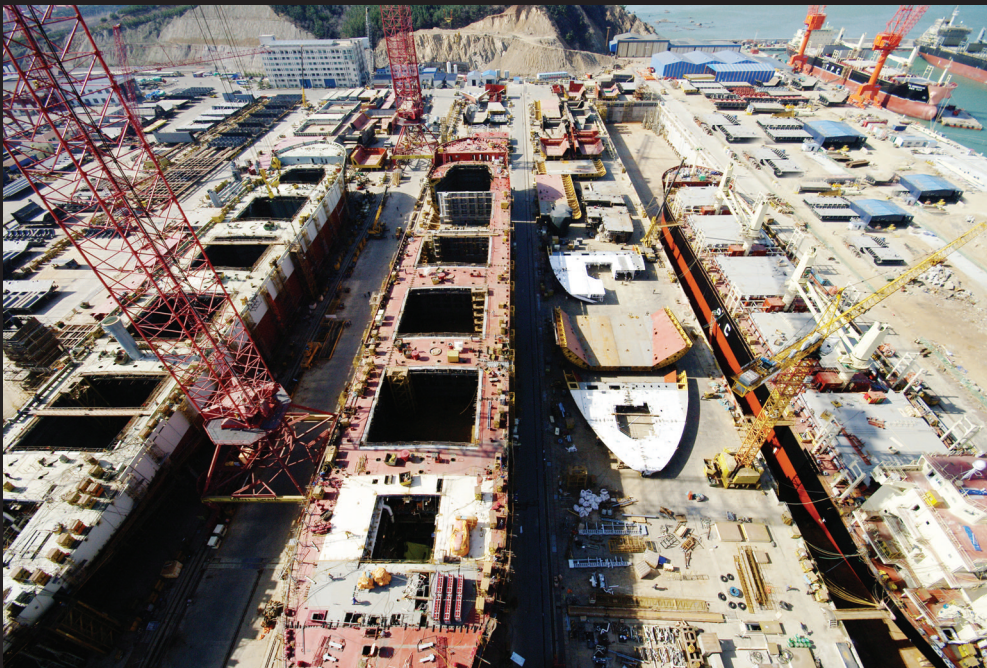
Outside view of the No. 1 factory
