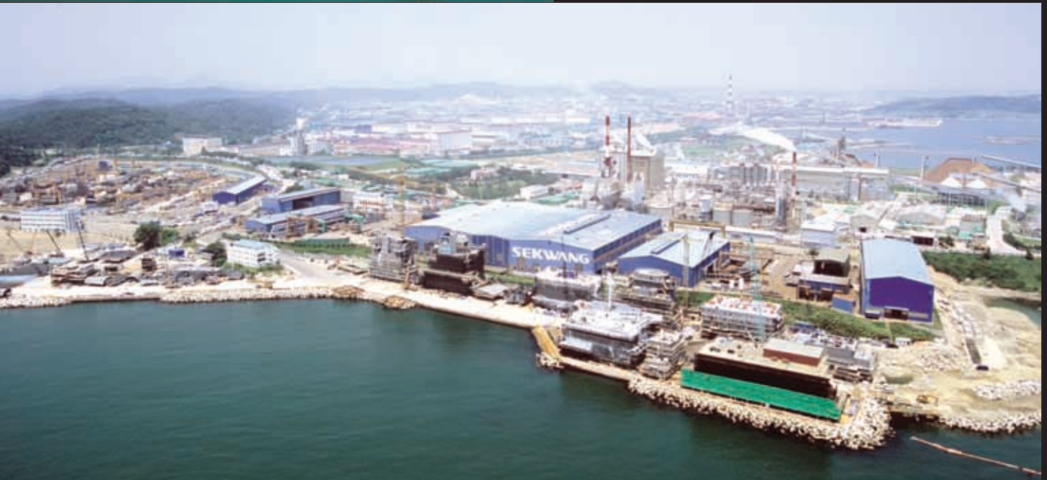
View of the No. 1 and No. 2 factory in the headquarters (main shipyard) of Sekwang Heavy Industries
