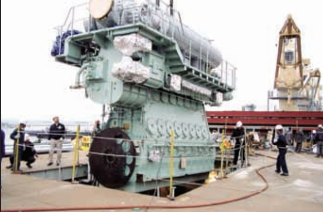
H1111 18,200DWT bulk carrier engine being installed (ship owner: VOSCO, Vietnam Ocean Shipping Joint Stock Company)
